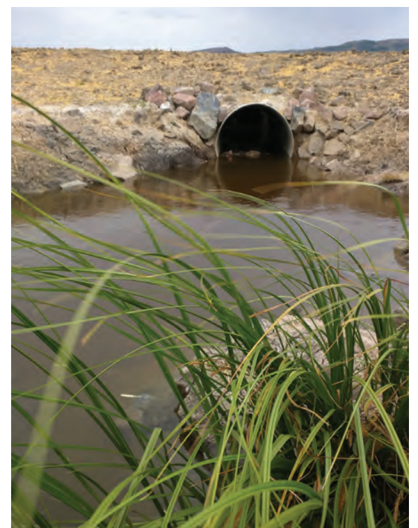
Structure at Lake Creek enhances water delivery.
