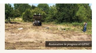
"For the restoration, we installed a low berm to impound water, similar to a beaver dam," said Matt Hough, DU conservation programs manager for Kansas. "We installed a water-control structure, removed invasive trees and excavated sediment to restore the natural depth of the wetlands."
