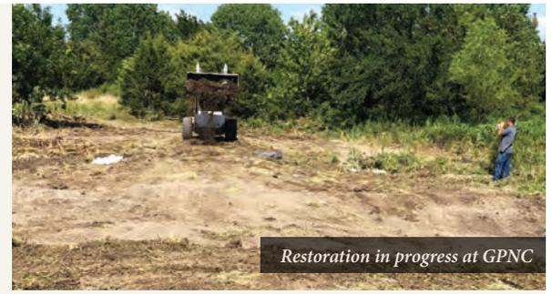
“For the restoration, we installed a low berm to impound water, similar to a beaver dam,” said Matt Hough, DU conservation programs manager for Kansas. “We installed a water-control structure, removed invasive trees and excavated sediment to restore the natural depth of the wetlands.”
