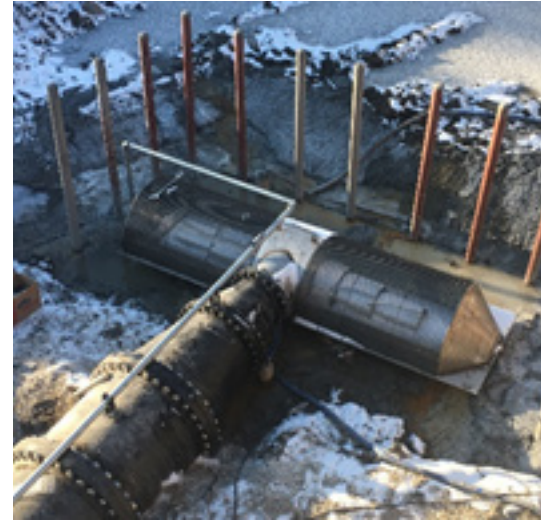
Water pump with protective screen installed on Neosho WA. The pump is surrounded by steel bollards that block large debris that could damage the pump.
