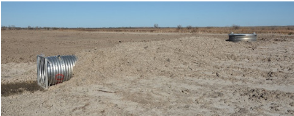
Water control structure will regulate water levels in wetland impoundment on Talmo WA.
