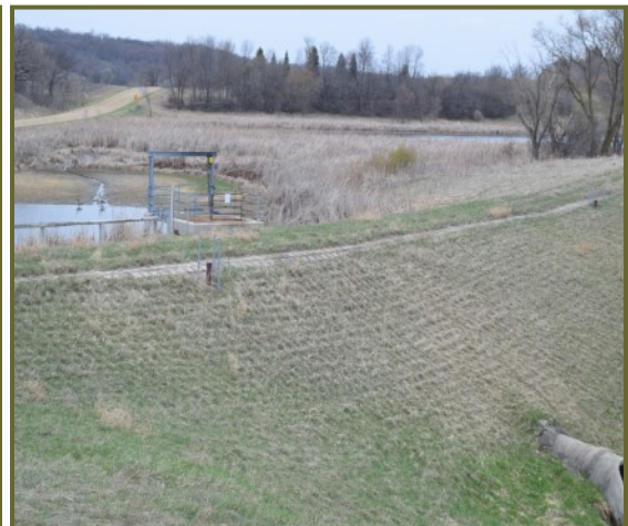
Above: A view of the 16-foot high dike and water control structure constructed in 1996 to restore the Stang Lake shallow lake basin.
