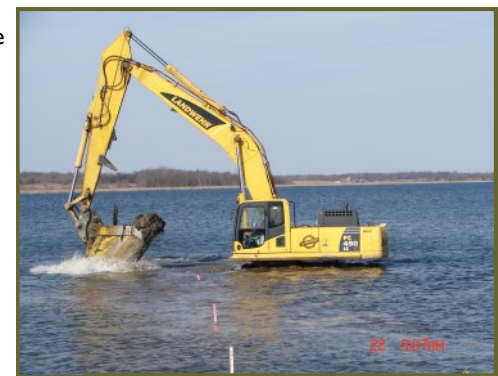
Above: A backhoe works out into the lake to dig a channel to the outlet.
