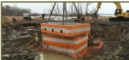
The lift station required several precast sections being lowered into place on the lift station base.
