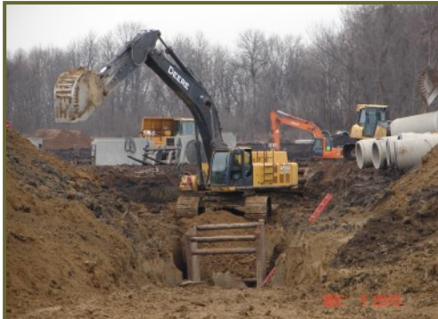
Above: Backhoes work to install the new outlet route for the lake.
