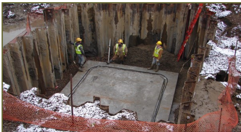
Left: The base of the large pump station needed to be installed several feet into the ground.
