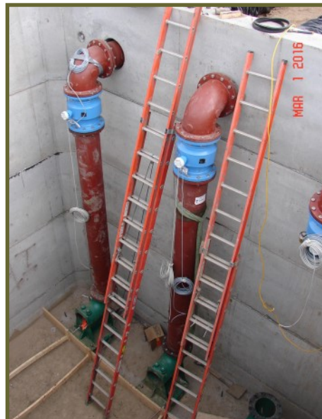
The interior of the lift station as the pumps and piping are being installed.
