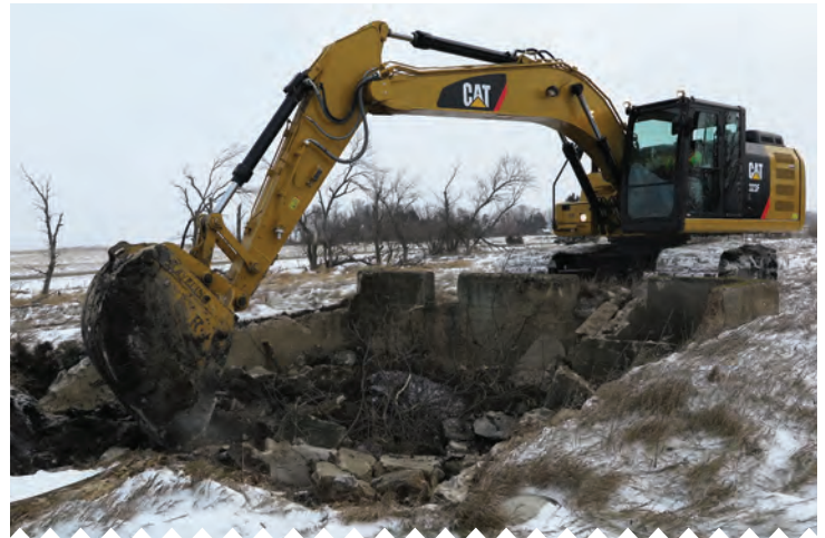
Excavating a depression and filling a drainage ditch to hold water in previously drained wetlands.
